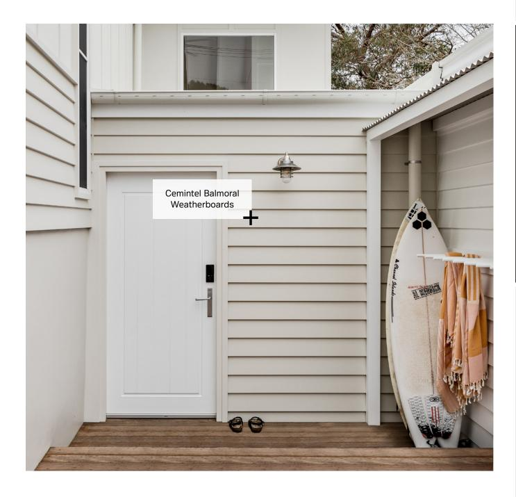
Balmoral Weatherboards have a 16mm thick profile providing sharp lines with a distinct shadow. Balmoral is pre-primed and ready to paint. It is lightly textured to give an even paint finish. The planks have a concealed fixing system and a tongue and groove profile so the boards easily slide together and provide a flat surface finish.
