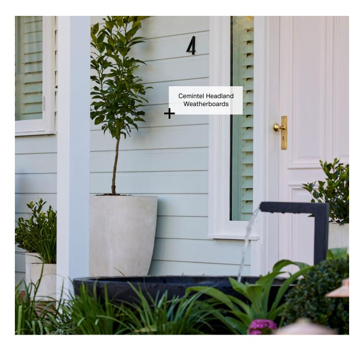
The weatherboard has a 25mm overlap which conceals fixings and they are gun nailable. This profile is fixed in a ship-lapped manner and is simple to install.
