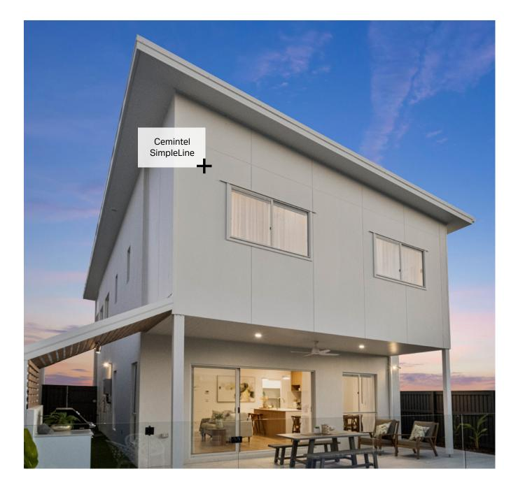
The Australian manufactured panels have shiplapped vertical edges that are suitable for gun-nailing for fast installation. There are multiple installation methods to give you choice and flexibility including direct fix or ventilated cavity options.
