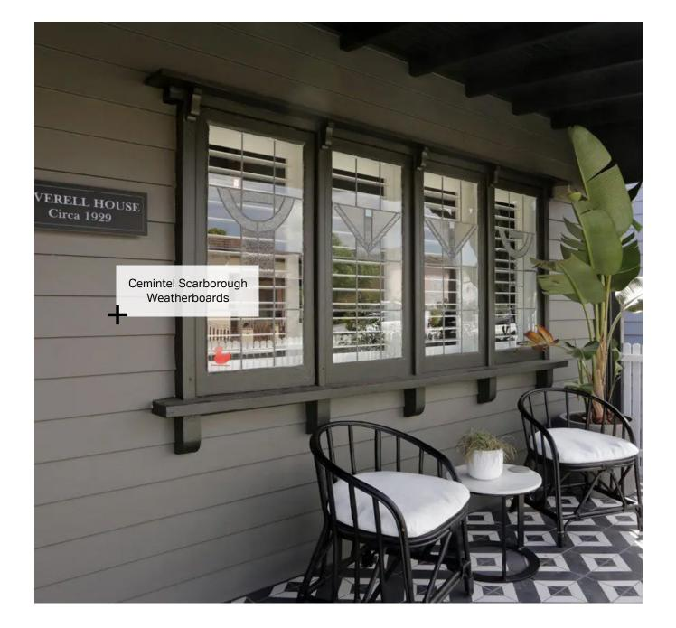
Scarborough® has a concealed fixing system and square profile so the boards butt together and provide a flat surface finish. The pre-primed boards are also able to be cut at different lengths to minimise waste. The nail groove reduces the thickness to 8mm for ease of nailing and keeping accuracy.
