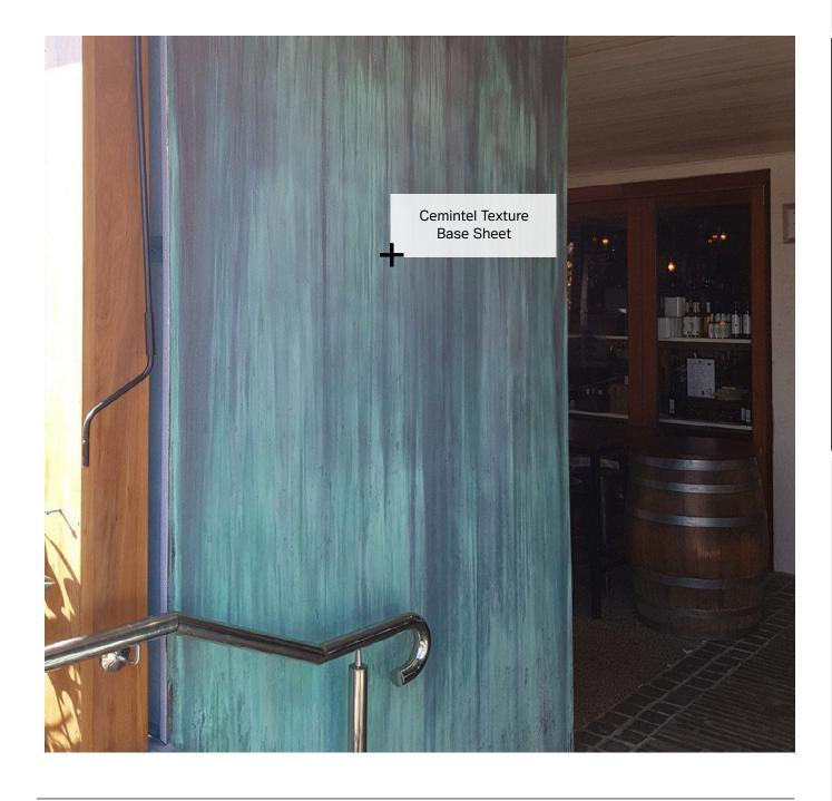
Texture Base Sheet is 7.5mm thick, with recessed edges for flush jointed external walls. When properly installed using the proprietary jointing, framing and coating system, Texture Base Sheet enable the creation of a seamless, weather resistant facades. They can be direct fixed or cavity fixed to create a ventilated and drained cavity system.
